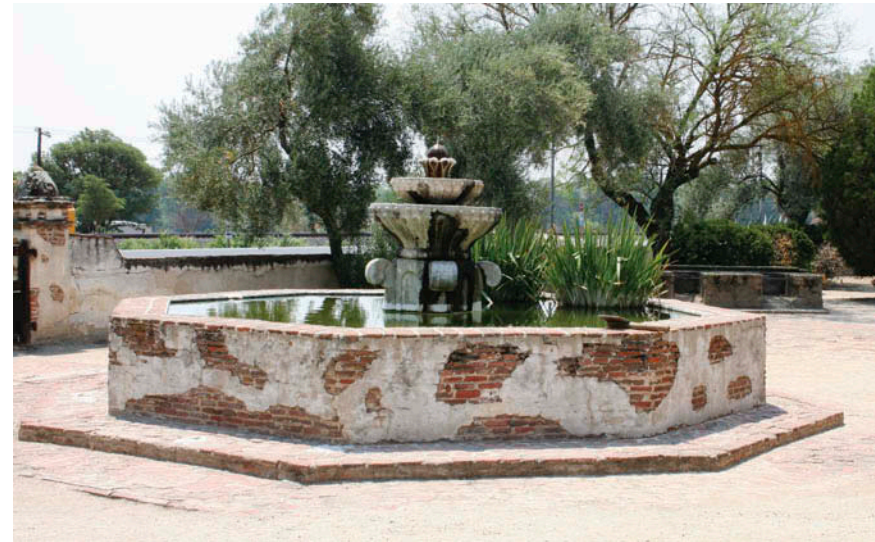
FIGURE 2. Fountain at Mission San Miguel with a treatment simulating failing stucco over adobe bricks. Source: photograph by the author. Permission to reuse must be obtained from the rightsholder.
