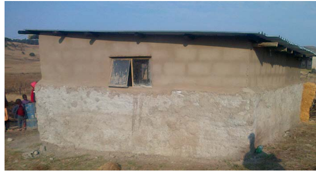
Figure 15: Completed Side Elevation
