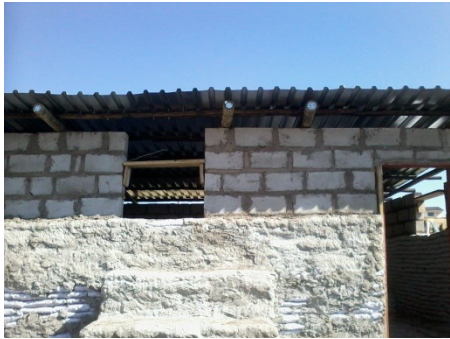
Figure 14: Completion of the Roof
