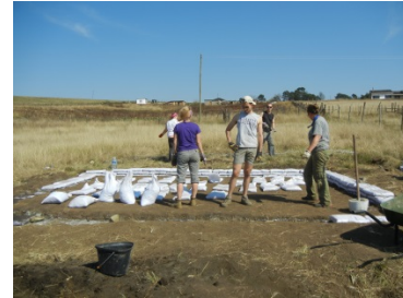
Figure 11: Building the Walls
