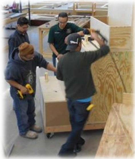
Figure 2: Building the Prototype
