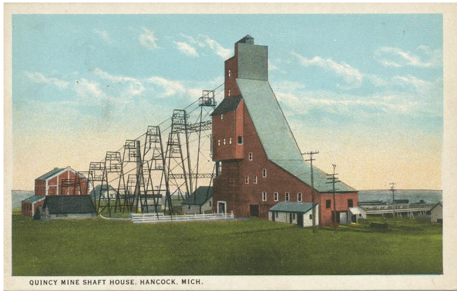
Figure 4. Postcard depicting Quincy Mine Company shafthouse No. 2 in the foreground and the hoist house behind it. Steel towers carry cables on pulleys from the hoist house to the shafthouse. The shaft had a length of 9,260 feet with a vertical depth of 6,225 feet.
