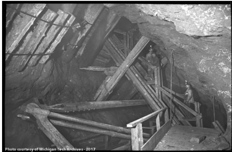
Figure 2. Photograph showing the Quincy Mining Company man-engine from the side. Platforms are spaced 10 feet apart. Two miners on the near platforms are going up, while the miner on the far platform is heading down the shaft. (Michigan Technological University Archives -ACC 239-5-6-1985-02-90)
